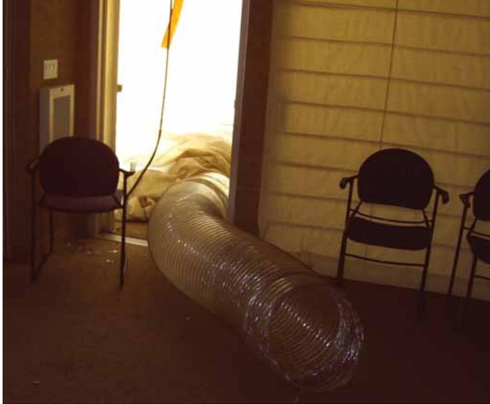
The size and type of heater used varies depending upon the layout of the building and scope of the problem. The only constants are the need for containment and filtration.
